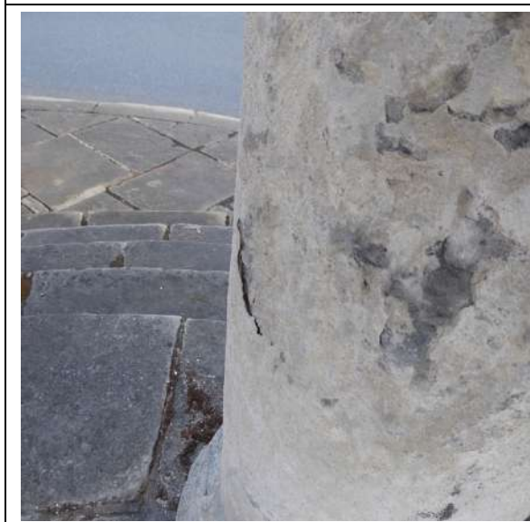
Column 3: The modern surface coating/repair layer is starting to come away on the inside. This needs to be lightly scaled
