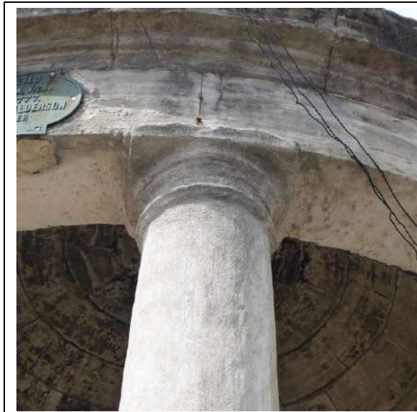
Column 1: Detail of column head. Iron pins in the tintol joint discussed later
