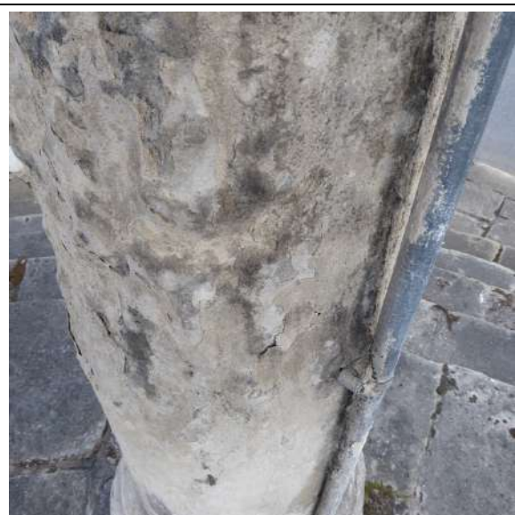
Column 3: The modern surface coating/repair layer is starting to come away on the inside. This needs to be lightly scaled
