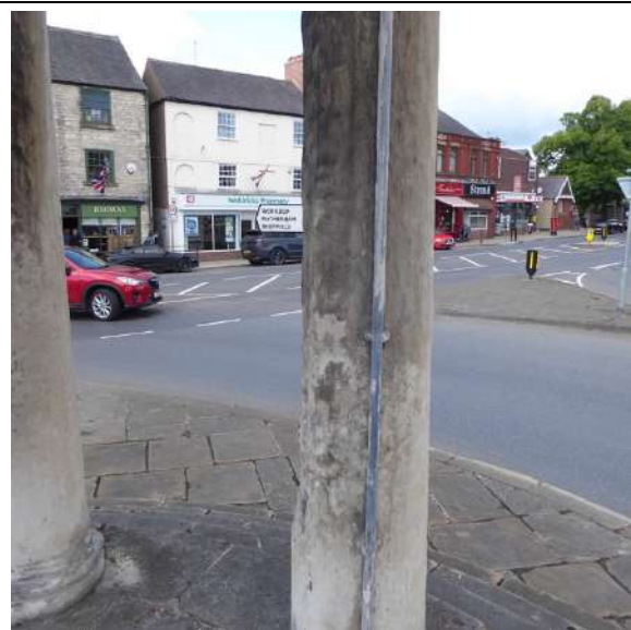
Column 3 (North): General views. This column has the conduit for the electrical feed.
