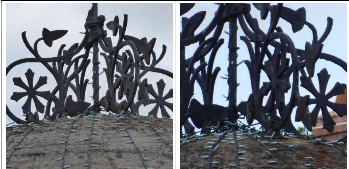
Weathervane: Photos showing loop staples which must be the main fixing we suspect these are set in lead.
