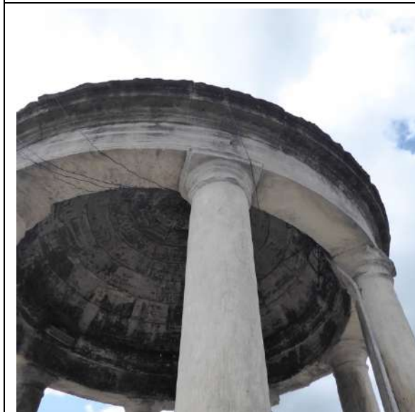
Column 1: Detail of column head. Iron pins in the tintol joint discussed later
