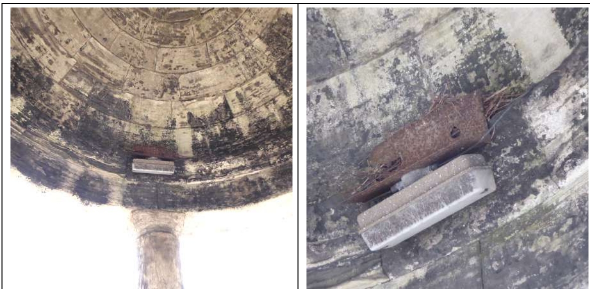
Light fitting at the south side is corroded and hanging off its bracket. Creates good nesting opportunity
