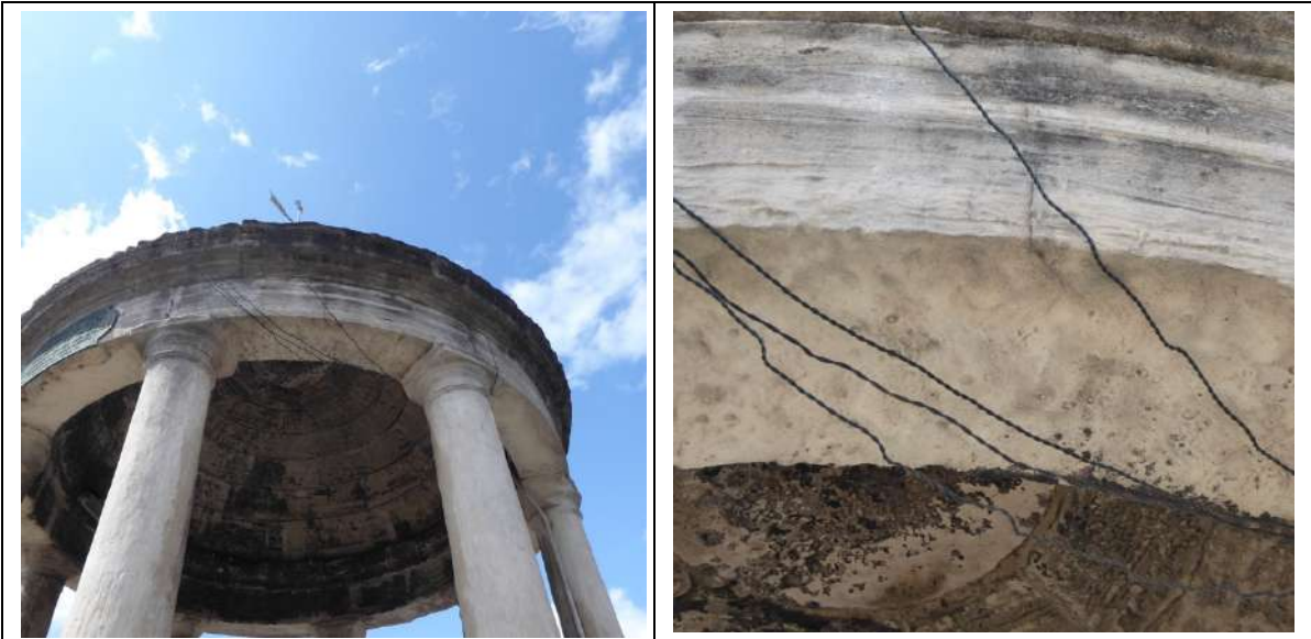
Lintel 2. Possible small crack in the soffit edge. The edges of this are weathered and dirty suggesting it is an old defect. This may be a clay seam defect in the stone rather than an actual crack. This should be monitored.
