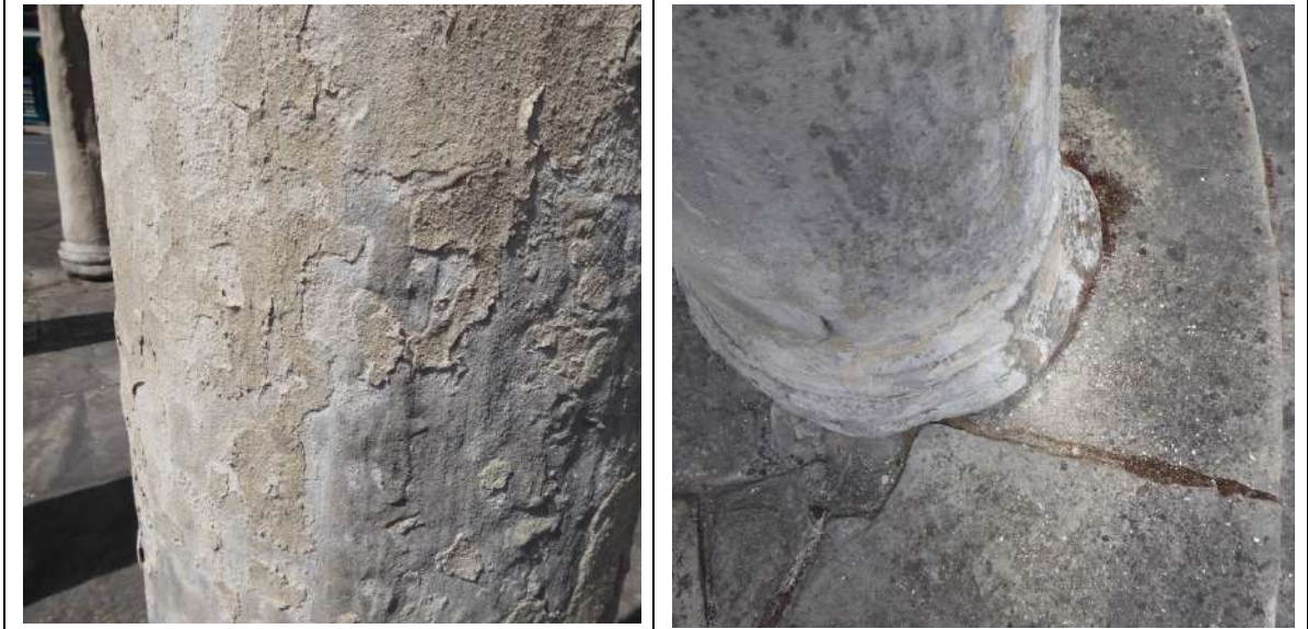
Column 1 (East): Past overcoating of a soft paint can be rubbed away. This may be a soft lime shelter coat which is a good product and should be repeated. If past specifications can not be found to confirm on the material used it may need to be teseted in a lab.
