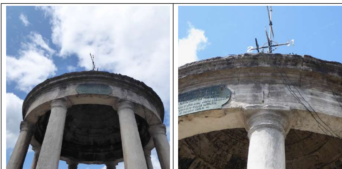
Lintel 1 (East). Showing the general arrangement. Photo also shows the 'nibbled edge' of the encircling cornice. This could be re-defined as a circle by adding a blade of lead into the joint above. It would also help the water drip clear of the
