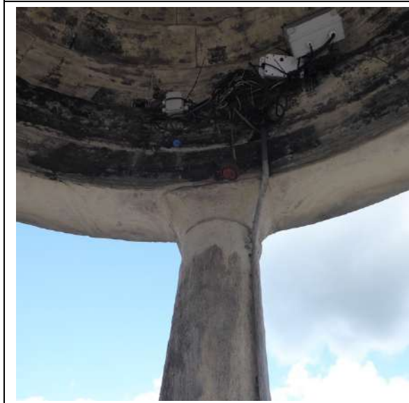
Column 3 (North): General views. This column has the conduit for the electrical feed.
