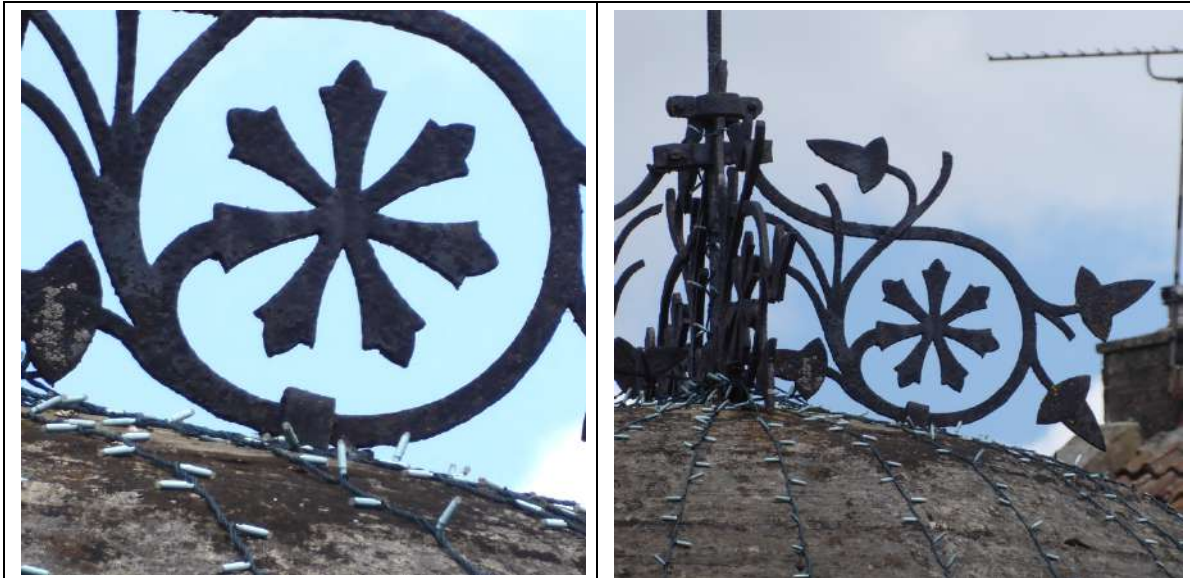
Weathervane: Photos showing loop staples which must be the main fixing we suspect these are set in lead.
