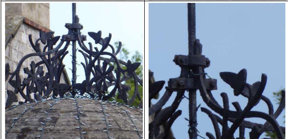
Weathervane: Photos showing the central rod. It is unclear if this is set into the stone or just clamped by the rest of the
